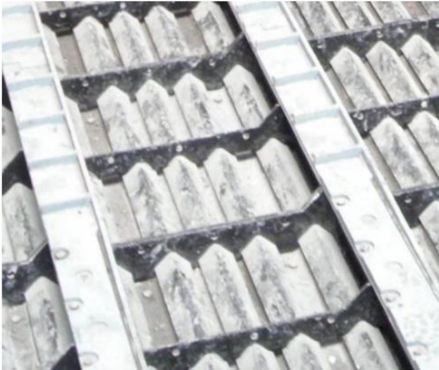
Aeration Cassettes at the time of erection in 2007
