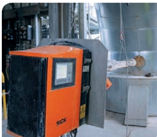
Left - Figure 2: Installation of the GM32 at the SCR inlet at the Geseke plant.
