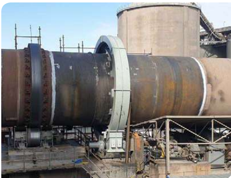
Below: The completed repair.
