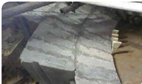
Left: The lining of the preheater inlet arch in 2014.
