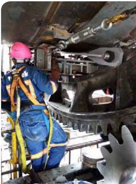
Above: Working in a confined space under the kiln.
