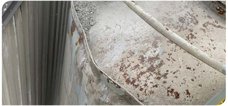
Above: A silo bulge is a serious indication of over-pressurisation within the silo and should not be ignored.
