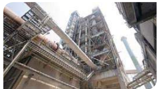
Below: One of Cimenterie Nationale's three preheater towers. Source: Cimenterie Nationale website.
