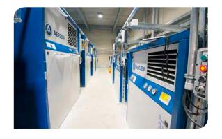
Left: A machine park consisting of AERZEN Delta Hybrid and Delta Blower provides the process air. Source: www.sienk.de.
