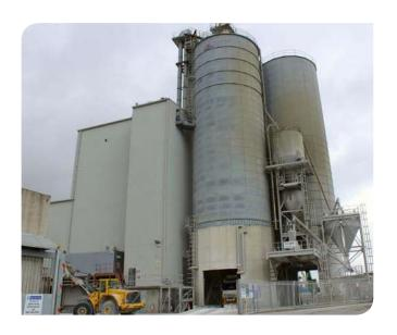
**Right:** The Ecocem grinding plant in Dublin was the first facility to supply GGBS to the Irish market in appreciable quantities. It can produce 0.35Mt/yr of GGBS.
