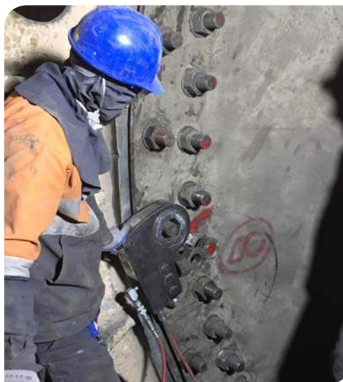
Left: Tightening the fixation bolt of the new trunnion with a torque wrench spanner.
