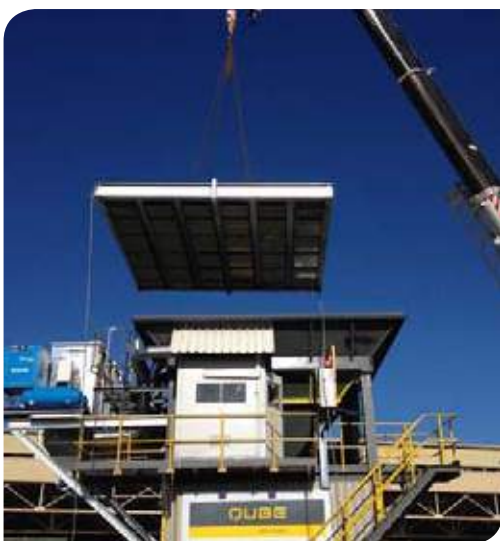
Below right: On-site checks ahead of the installation.
