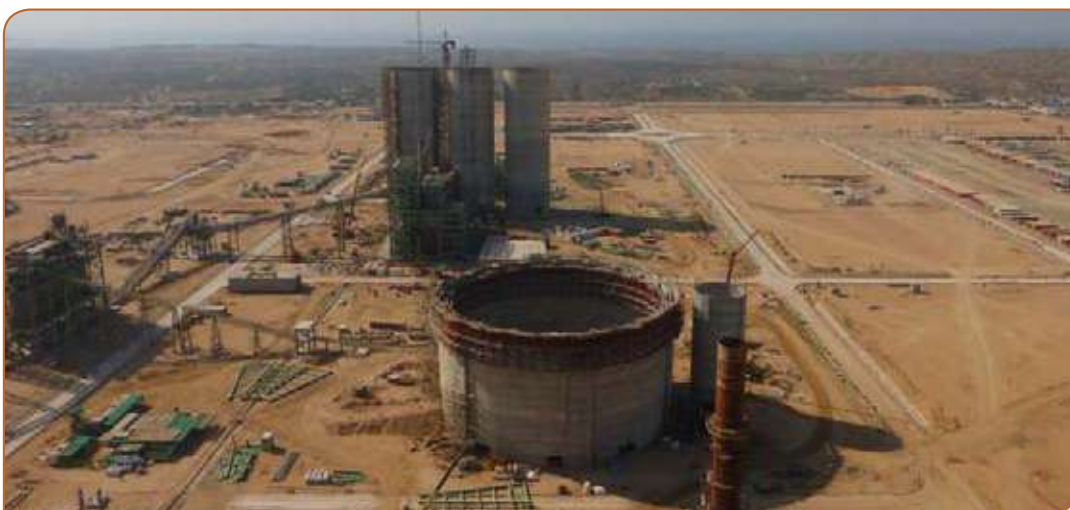
Right: The Hub plant's clinker and cement silos under construction, with the shoreline of the Arabian Sea just visible in the far distance.
