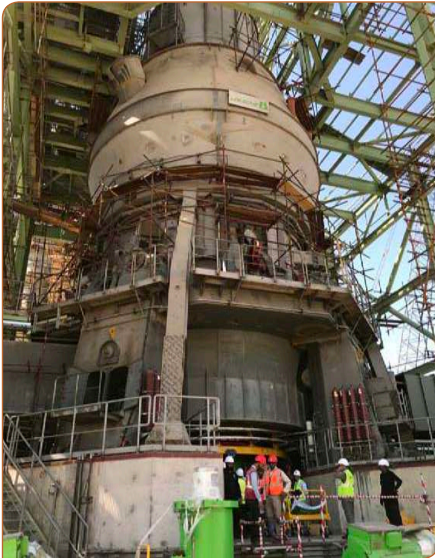
Above: The world's largest raw materials grinding mill, under construction at the Hub cement plant project site. The 654t/hr raw mill from Loesche features a COPE drive from RENK.
