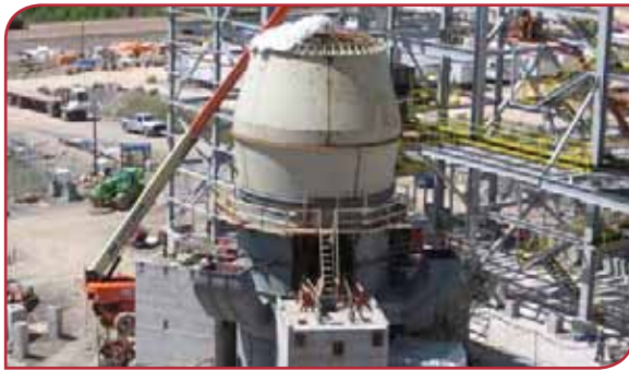
Above: Installation of a finish mill at McInnis Cement. Source: McInnis Cement website.
