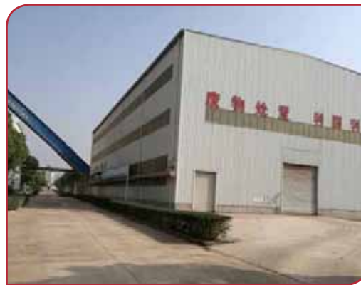
Left - Figure 3: Exterior view of the waste sorting plant.
