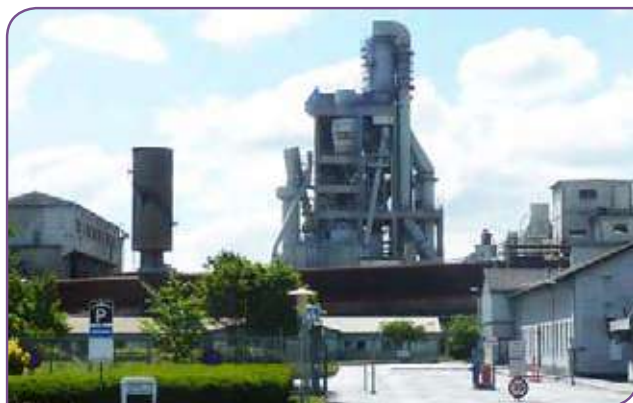
Above: Preheater, with long kilns in the foreground. The Aalborg site has seven kilns in total.
