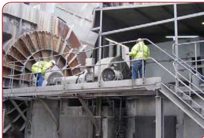
Right: Siemens engineers carrying out an inspection prior to conversion to an integrated drive systems (IDS) solution.
