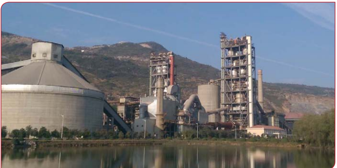
Below - Figure 1: The Anhui Conch Xuancheng plant in Anhui Province, China has recently had two electrostatic precipitators upgraded by Babcock & Wilcox.
