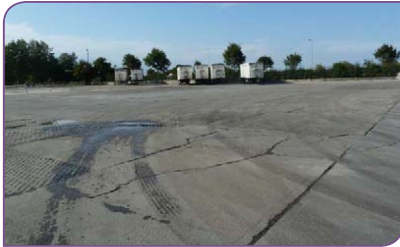
Left: A large area of ground has been cleared prior to construction of new office buildings for the plant. Work is expected to be completed by the end of 2017, four years since the flood.
