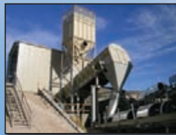
Truck Unloading Stations Receiving up to 1,200 t/h
