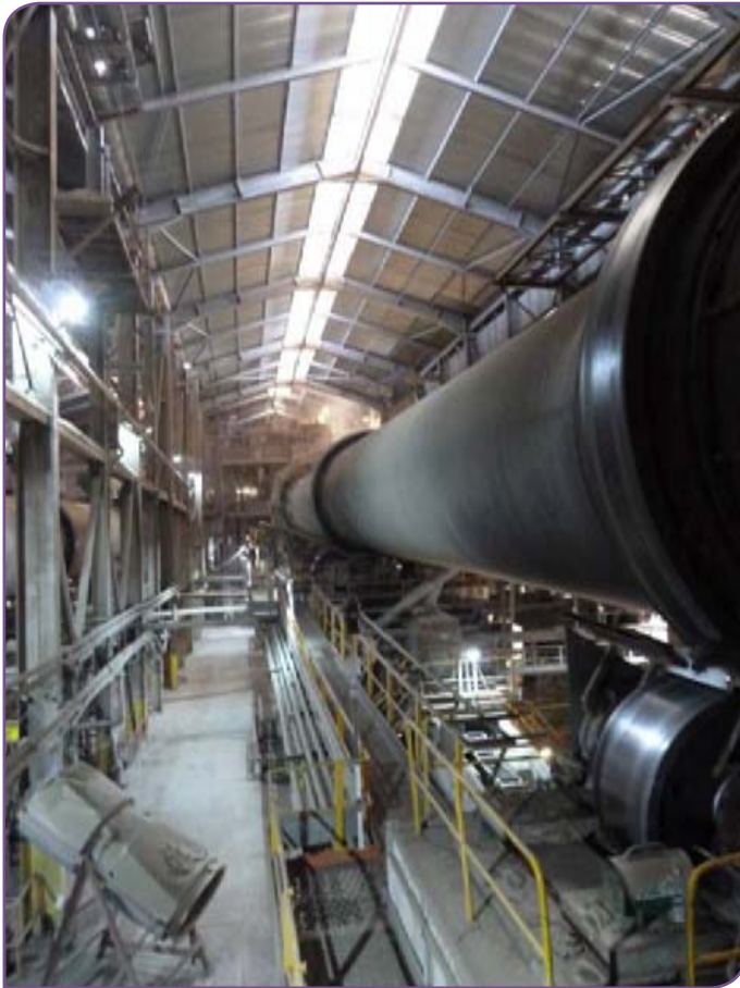
Above: Unusually, the two kilns at South Ferriby are covered.
