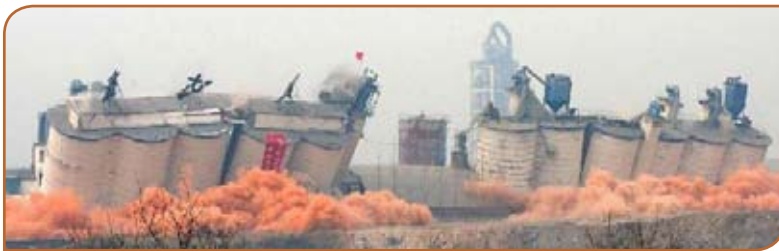
Below: Cement plant silos being demolished in Hebei Province in 2014.
