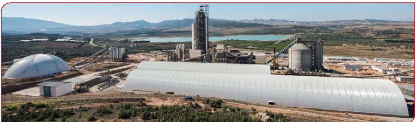
Below: Carthage Cement has Geometrica storage domes for Limestone, coal and additives.
