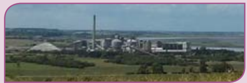
Above: The South Ferriby plant suffered the fire only months after the completion of renovation following extensive flood damage.
