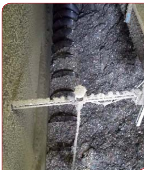
Left: Fill level measuring probes and other sensors monitor the automated processes.
