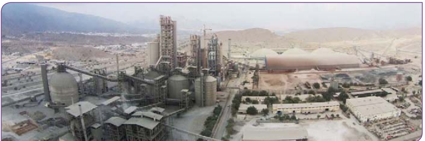
Below: The Oman Cement Company factory near Muscat, Oman is one of a number of Middle Eastern producers that has had to deal with increasing oil and gas costs recently.
