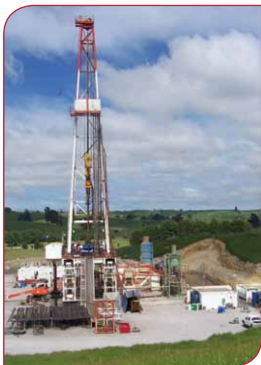
A Jacobs geothermal exploration drilling project in Wairakei, New Zealand. These kinds of projects are essential for researchers to find new and efficient methods of producing high-quality cement.
