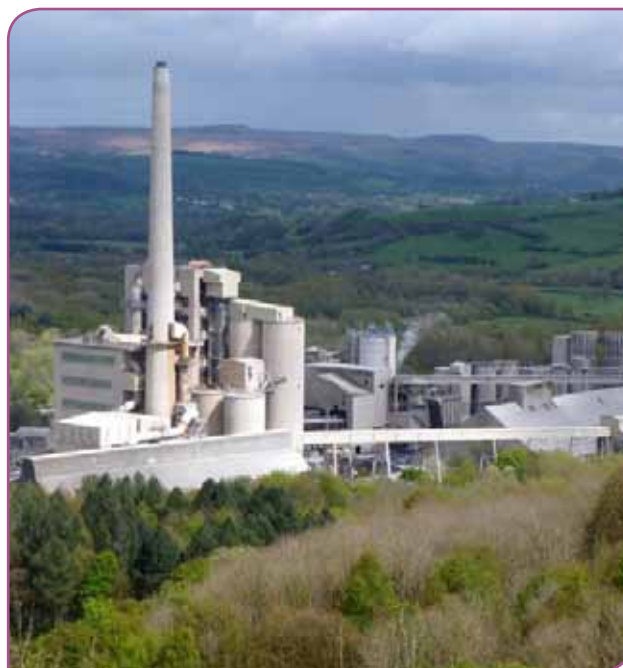
Right: The Hope Cement Plant in Derbyshire is one of the country's largest with a capacity of 1.3Mt/yr.
