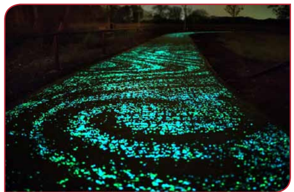
Above: A glow-in-the-dark cycle path, a potential application of José Carlos Rubio's glow-in-the-dark cement mixture. Source: Investigación y Desarrollo.
