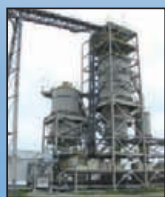
Silo Dischargers Discharging up to 1,000 t/h
