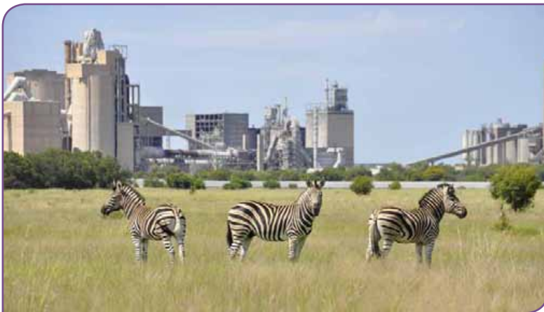
Above: The successful cement producers of the future will have to be more in tune with global sustainability needs.
