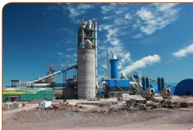
Left - Figure 7: The 1.1Mt/yr Jambyl Cement plant in Mynaral, Kazakhstan, which is 60% owned by France’s Vicat, plans to expand its capacity to 2.2Mt/yr with the addition of a new, duplicate cement line.
