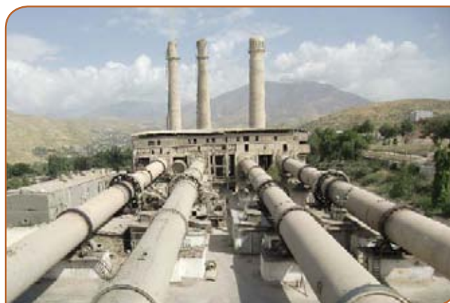
Right - Figure 12: The 1.1Mt/yr Tajikcement plant in Dushanbe, Tajikistan. Source: http://emagazine.european-times.com/tajikistan/industry-and-construction-tajikcement-transforming-tajik-raw-materials-into-world-class-cement
