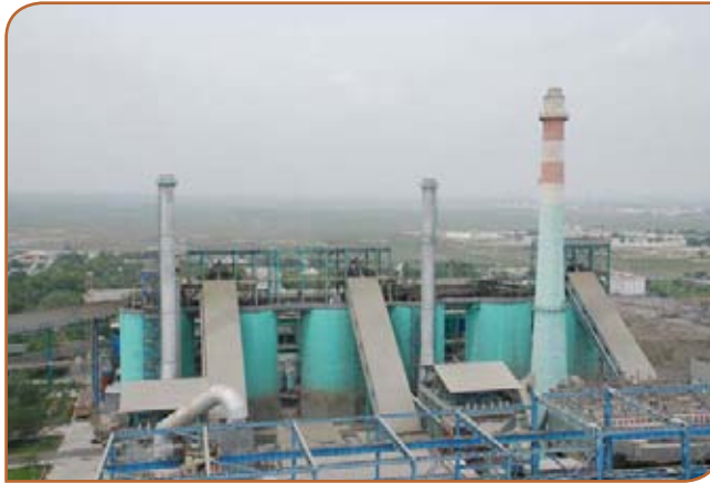
Right - Figure 16: The 3.08Mt/yr Qizilqumsement plant in Bukhara, Uzbekistan, is the largest in the country.
