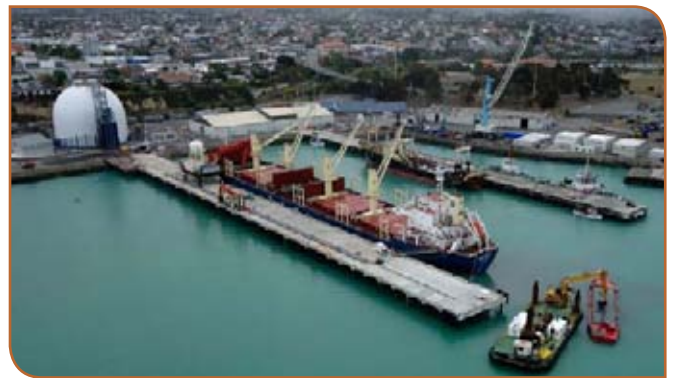
Holcim's first order of 22,000t of cement arrived at the Timaru Port in New Zealand via the Esperance Bay ship in December 2015.
