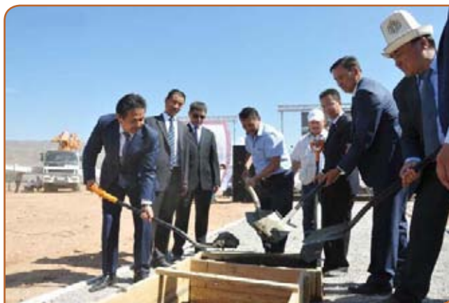
Right - Figure 9: Kyrgyzstan's First Vice Prime Minister Tayyrbek Sarpashev (far left) and Business Counsellor with the Chinese Embassy in Kyrgyzstan, Sun He (third from the right), attended the ground-breaking ceremony of the Zeth Cement plant in Kemin, Chui, Kyrgyzstan on 29 August 2014. Source: http://news.xinhuanet.com/english/china/2014-08/30/c_133606828.htm
