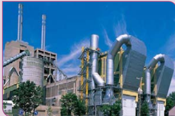
HeidelbergCement's Burglengenfeld plant will undergo a major modernisation project.
