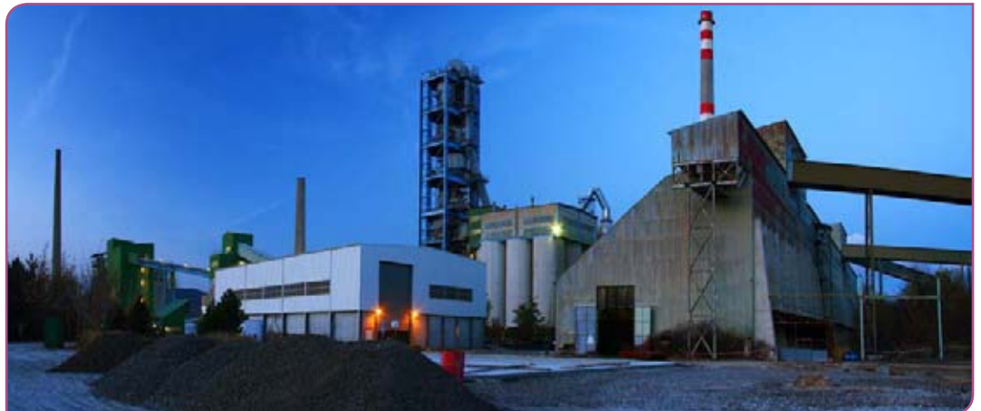
Right - Figure 6: LafargeHolcim's 1.1Mt/yr cement plant in Čížkovice. Learn more about the plant from Peter Edwards' plant visit report in this issue.
