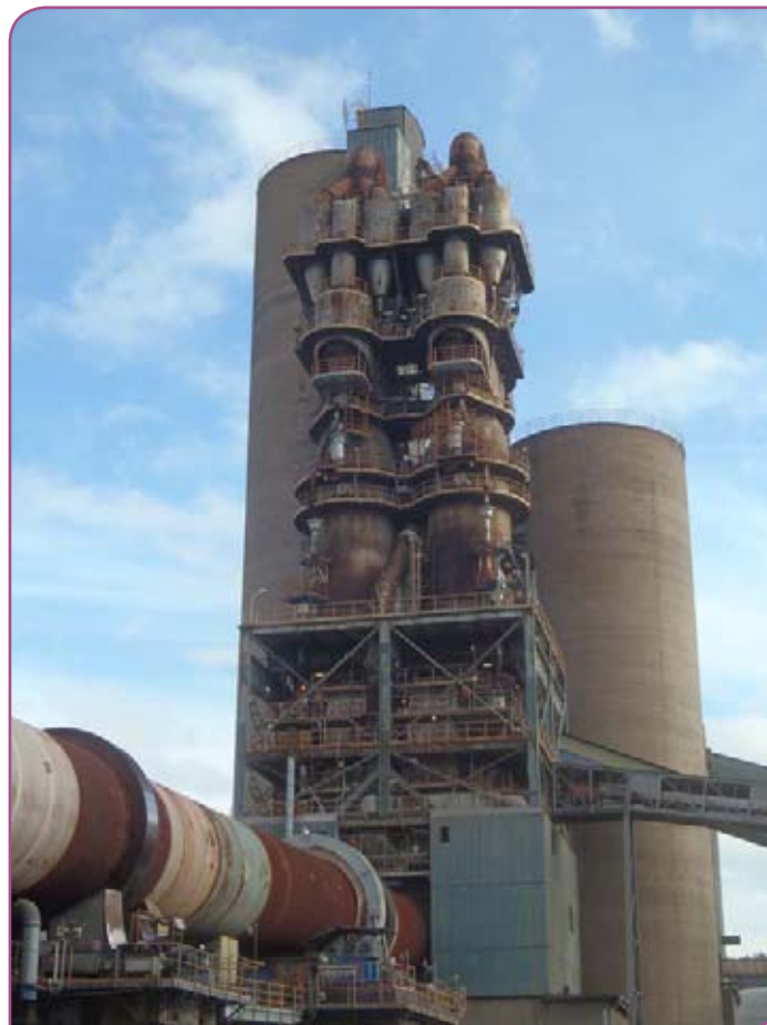
Left: View of the Prachovice plant’s preheater tower, an unusual one-and-a-half stage cyclone / shaft hybrid from PSP Engineering.
