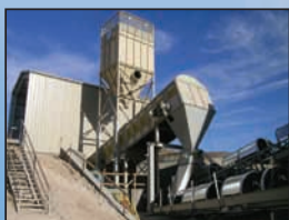
Truck Unloading Stations Receiving up to 1,200 t/h
