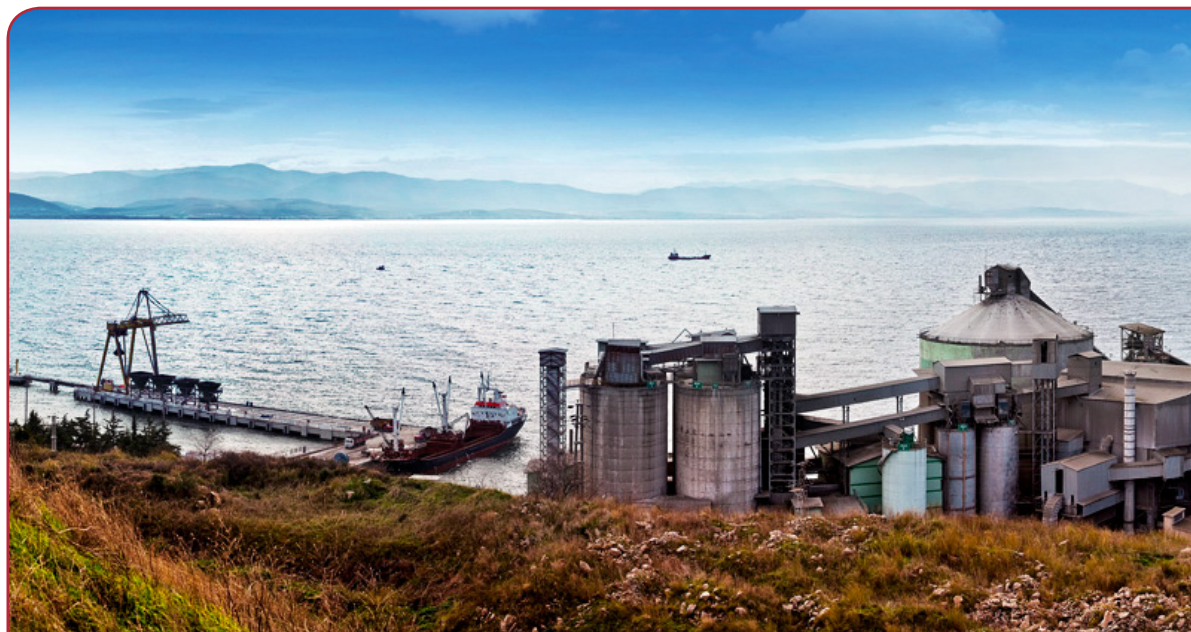
Right - Figure 1: The Aslan Çimento plant in Kocaeli, 30km from Istanbul, has 1.25Mt/yr of clinker and 2Mt/yr of cement production capacity.
