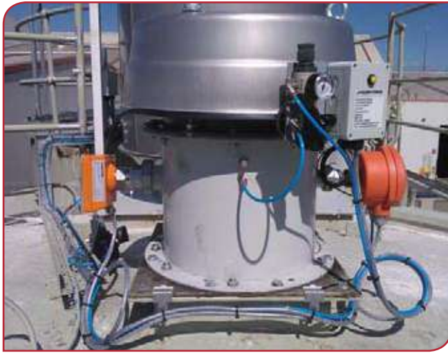
Above: Hycontrol recommends that the PRV, pressure sensor and high-level alarm be testable from ground level prior to every fill.
