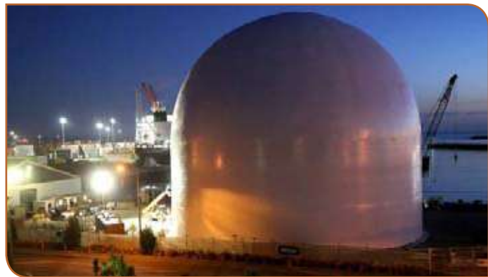
Holcim New Zealand's 30,000t cement silo on Auckland's waterfront in New Zealand.
