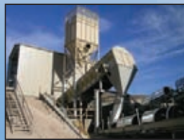
Truck Unloading Stations Receiving up to 1,200 t/h
