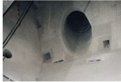
Heat resistant nozzle within brick work
