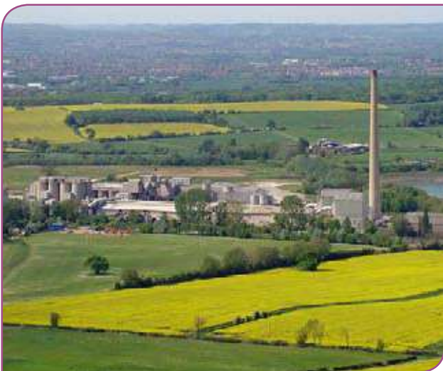
The Westbury cement plant in Wiltshire, UK, will be partly demolished.
