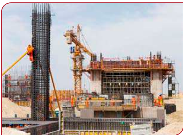
Cementos Pacasmayo's cement plant in Piura during the construction phase.
