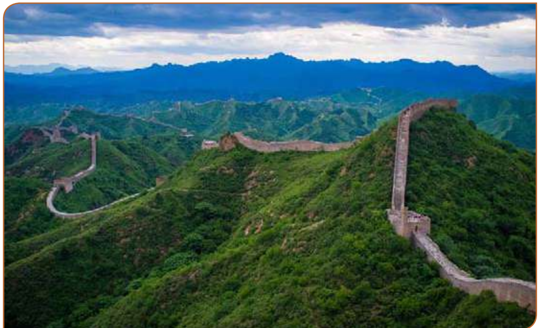
Right - Figure 1: The Great Wall of China at Jinshanling is a series of fortifications made of stone, brick, tamped earth, wood and other materials. It is built along an east-to-west line across the historical northern borders of China.
