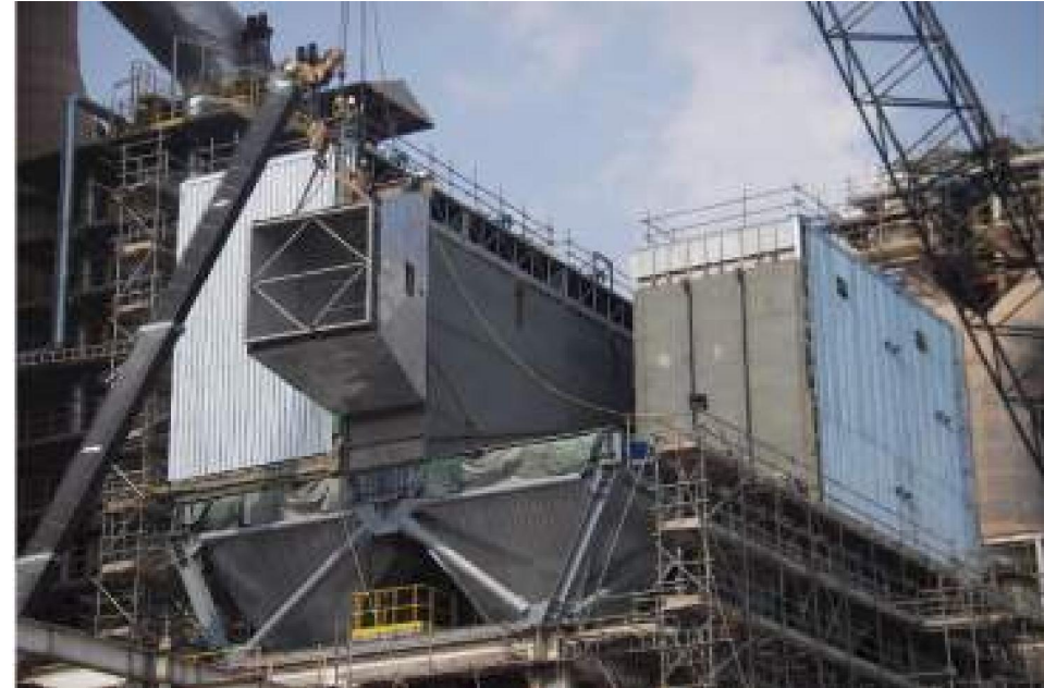
Kiln stack bag filter - 2013
