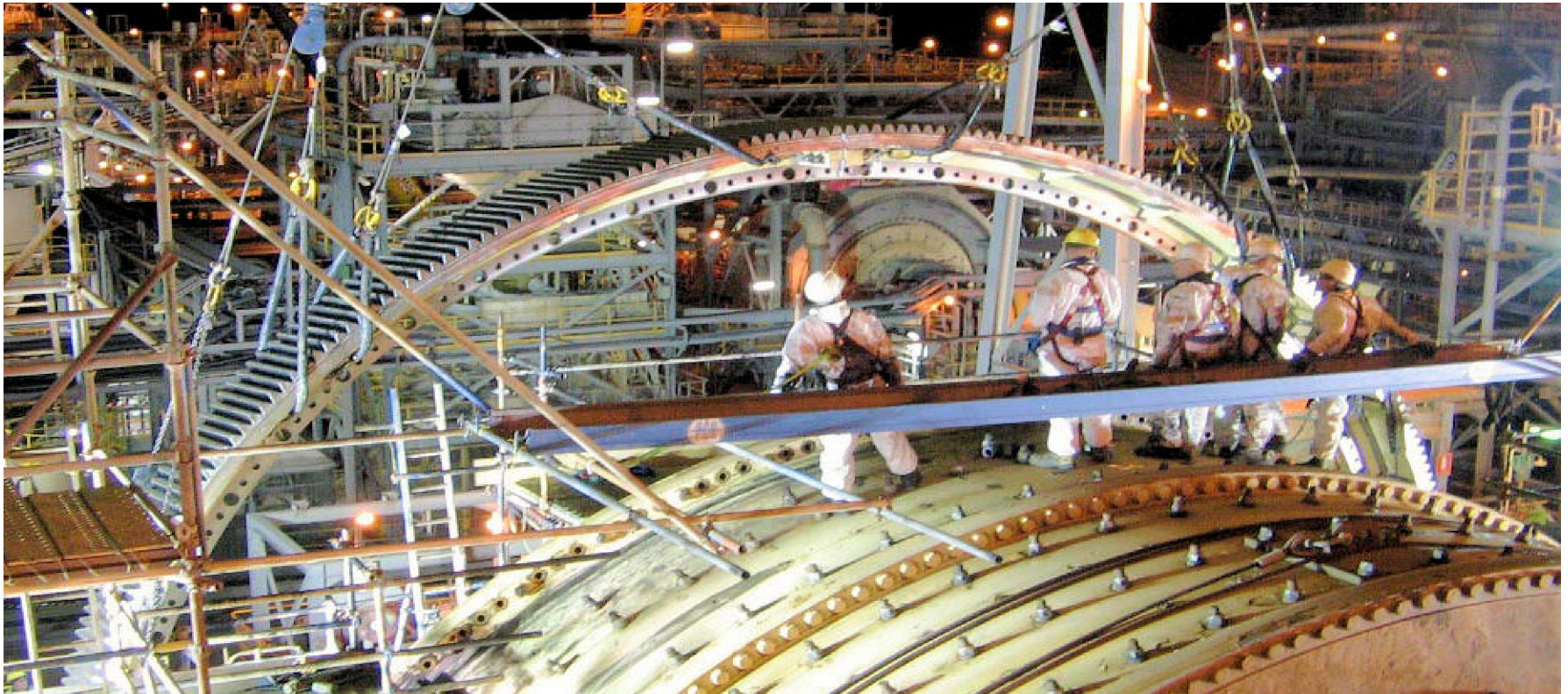
Installation of induction hardened 420BHN forged steel gear on 36 ft. (11.0 m) Mill (2006)
